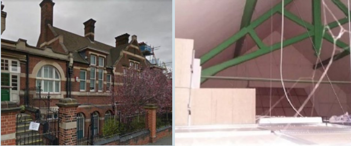
Figure 15: Example of a Victorian/Edwardian school roof
