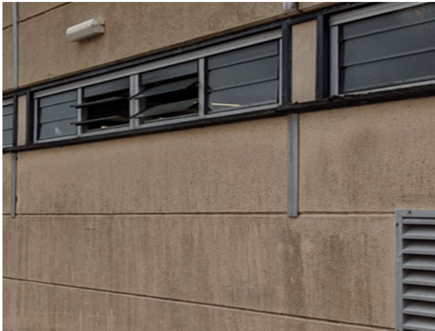
Figure 29: Exterior view of horizontal RAAC wall panels
