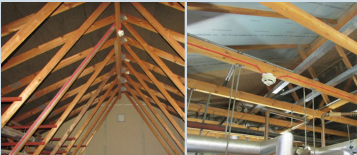
Figure 16: Examples of a modern timber roof
