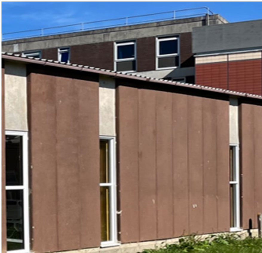
Figure 30: Exterior view of vertical RAAC wall panels
