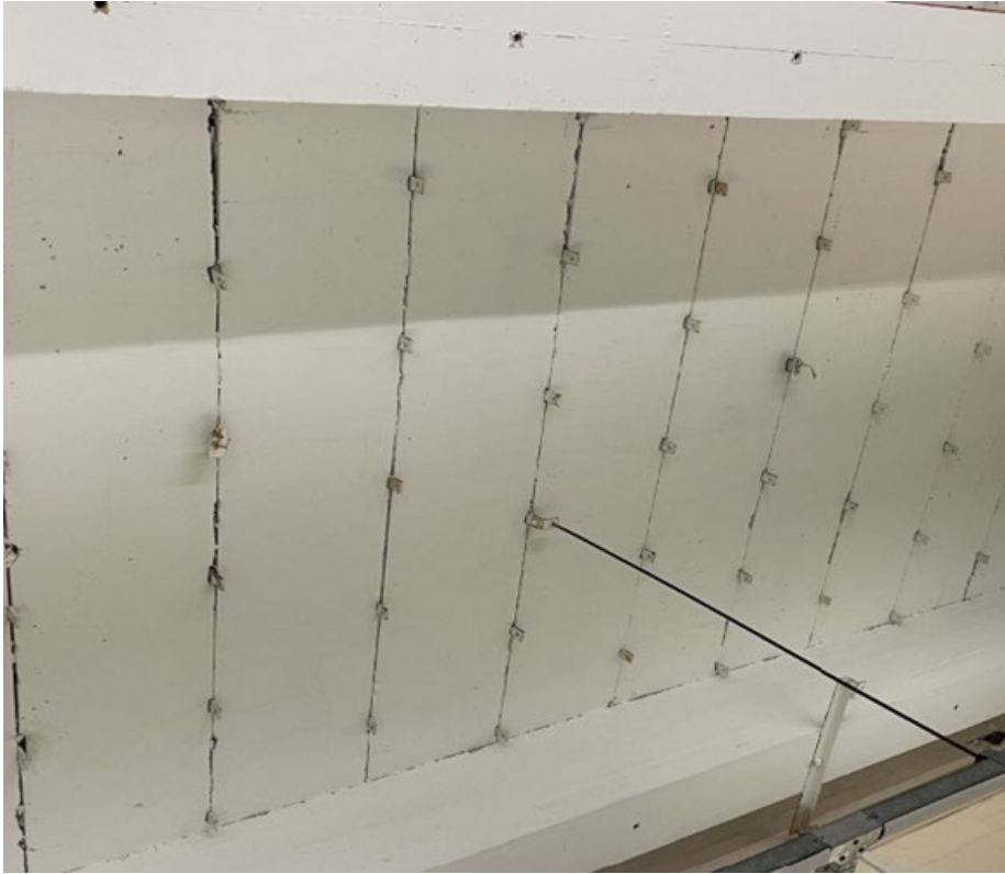
Figure 27: RAAC ceiling system with supports to services and suspended ceiling
