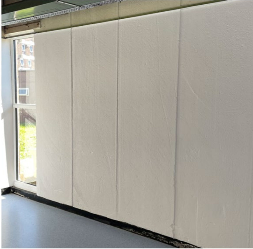
Figure 31: Interior view of vertical RAAC wall panels
