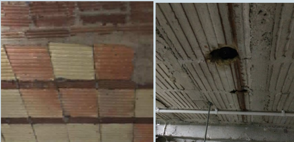
Figure 22: Examples of Beam and Pot Roofs
