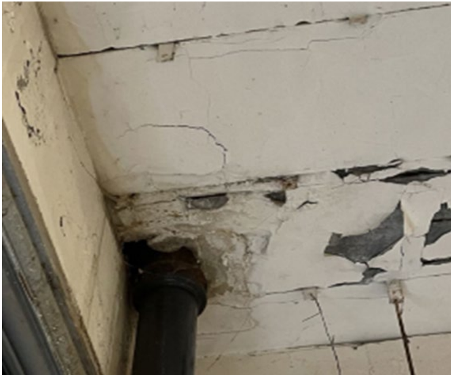
Figure 28: Example of adapted plank at services penetration
