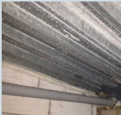
Figure 18: Example of a metal deck roof
